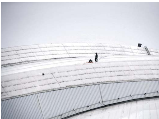
Building-maintenance workers examine a hole in the roof at Rogers Centre on Monday. The tear is believed to have been caused by a piece of ice that fell from the CN Tower. COLE BURSTON/THE CANADIAN PRESS
